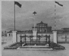
Spreequelle in Neu-Gersdorf
